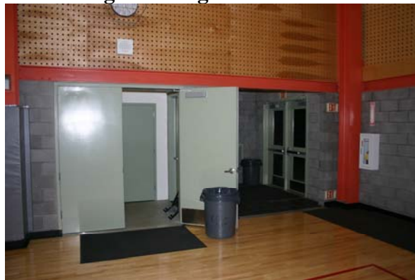
Egan Storage Room Door
